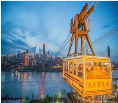
Changjiang Cableway 153 Xinhua Road, Yuzhong District
